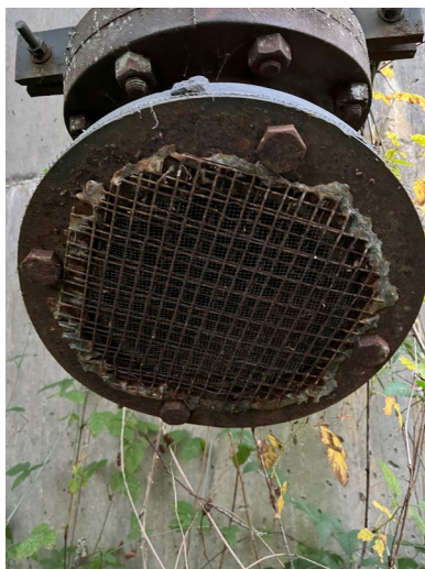
Figure 16. (Left). Cove Tank. Figure 17. (Middle). Screened overflow pipe. Figure 18. (Right). Hatch and gasket.
