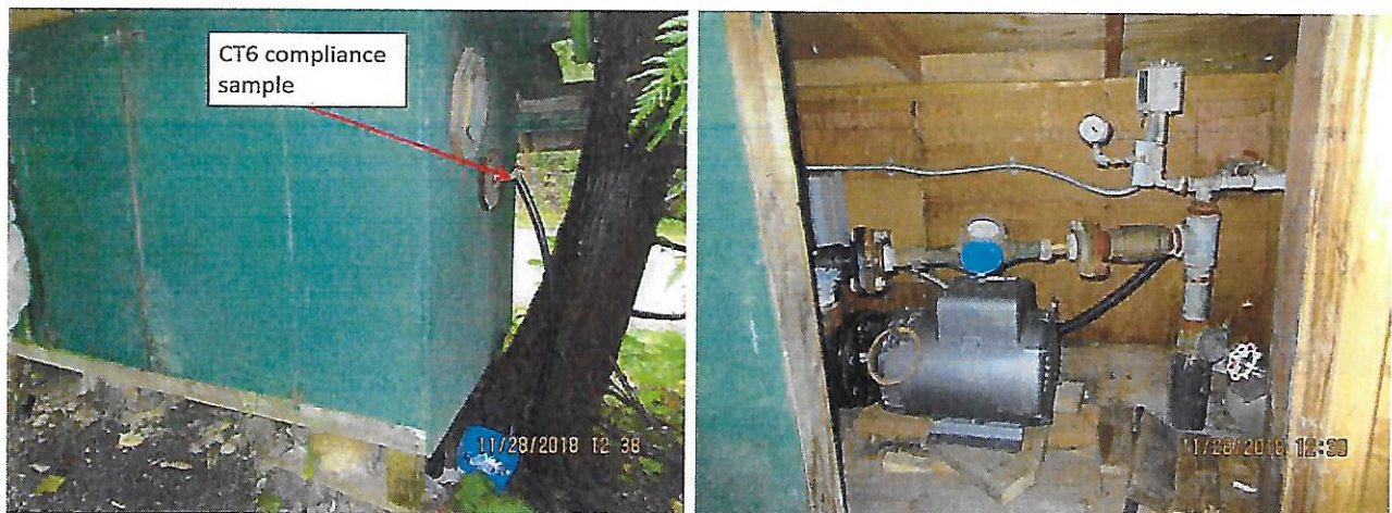
Figure 10. 156th Street BPS. (Left) Exterior view showing the entry point to distribution sample tap. (Right) Interior view.
