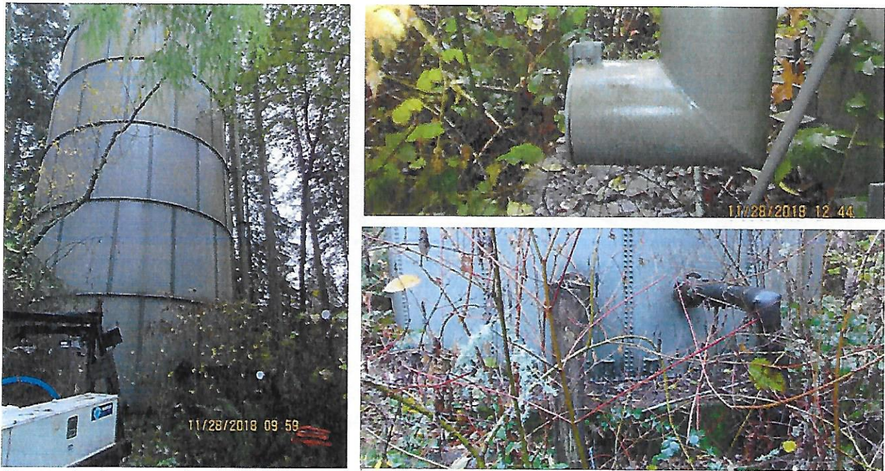
Figure 9. Green tank. (Left) Overview. Drain line daylights at roadside. (Right Upper) Exterior overflow with air gap and flapper valve. (Right Lower) Two inlets. Possible remnant of previous operation of the Green tank and Cove tank in parallel rather than series.
