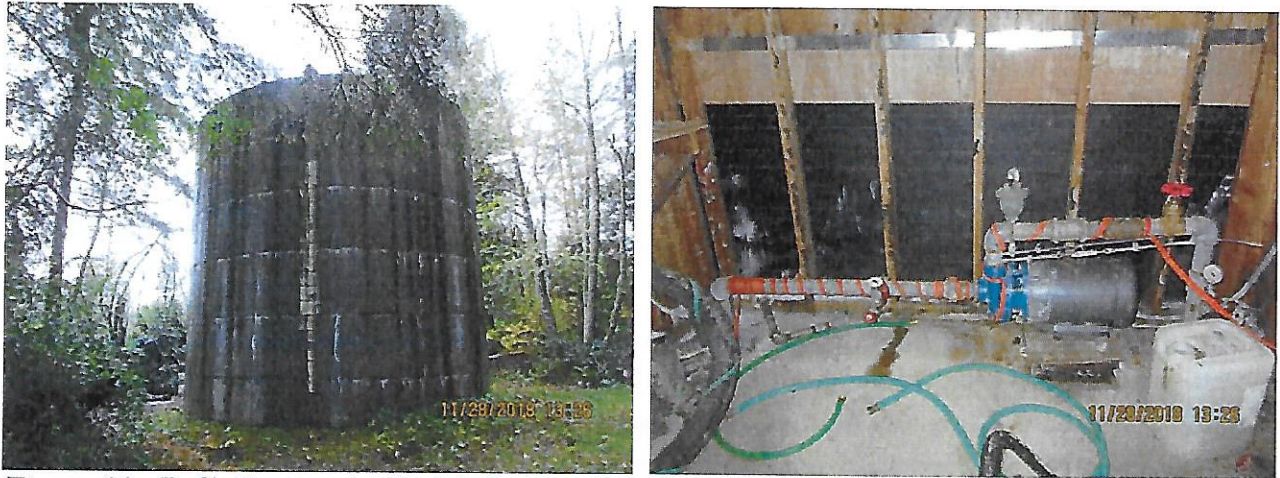
Figure 11. (Left) Cove tank. (Right) Cove tank PS. 65-psi discharge pressure. Please add a 24-mesh screen to the air-vacuum valve vent.
